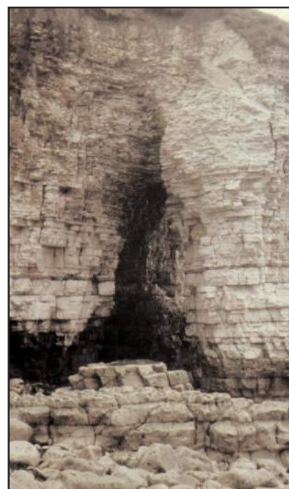
Figure 9: Taken only three months after the arch collapsed in 1984. Most of the debris has already disappeared
