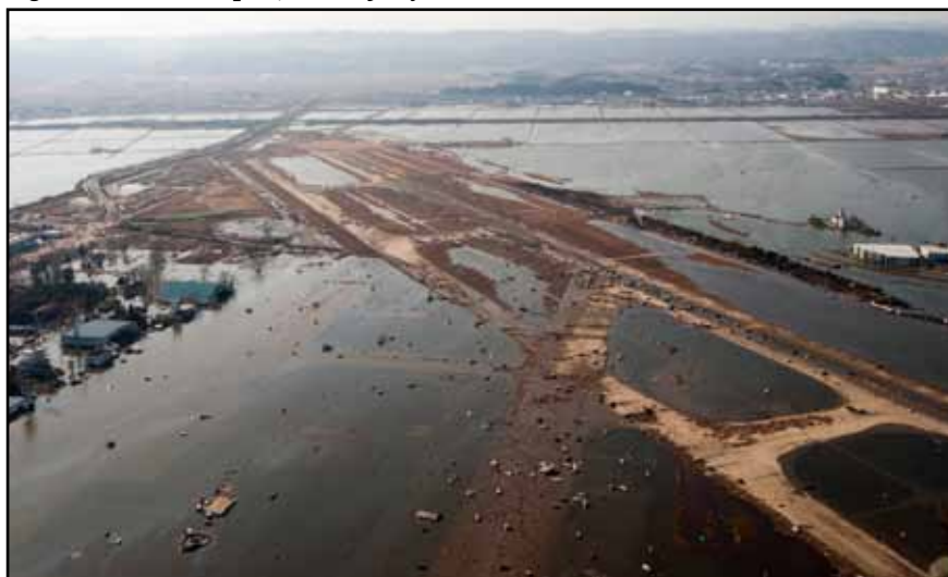
Figure 3: Sendai airport, two days after the tsunami
